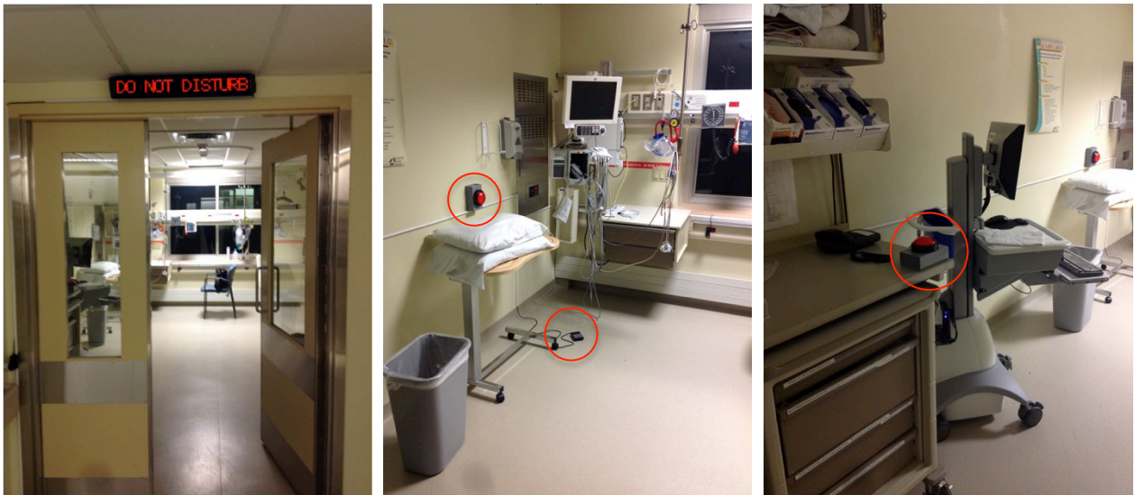
Figure 6. The installed LED sign (left), wall LED button and foot pedal (center), and the desktop LED button (right)
